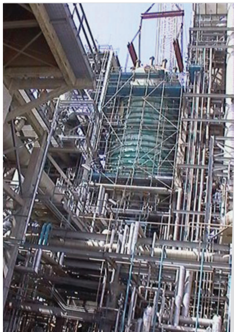
Diesel Hydrotreater Revamp EPC, Tulsa, OK
